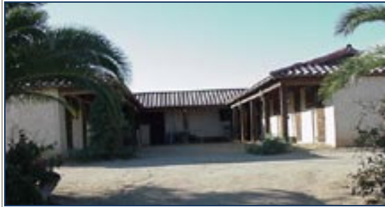
It took us one year of weekends to build this barn. Looking at the finished barn from the arena entrance.
